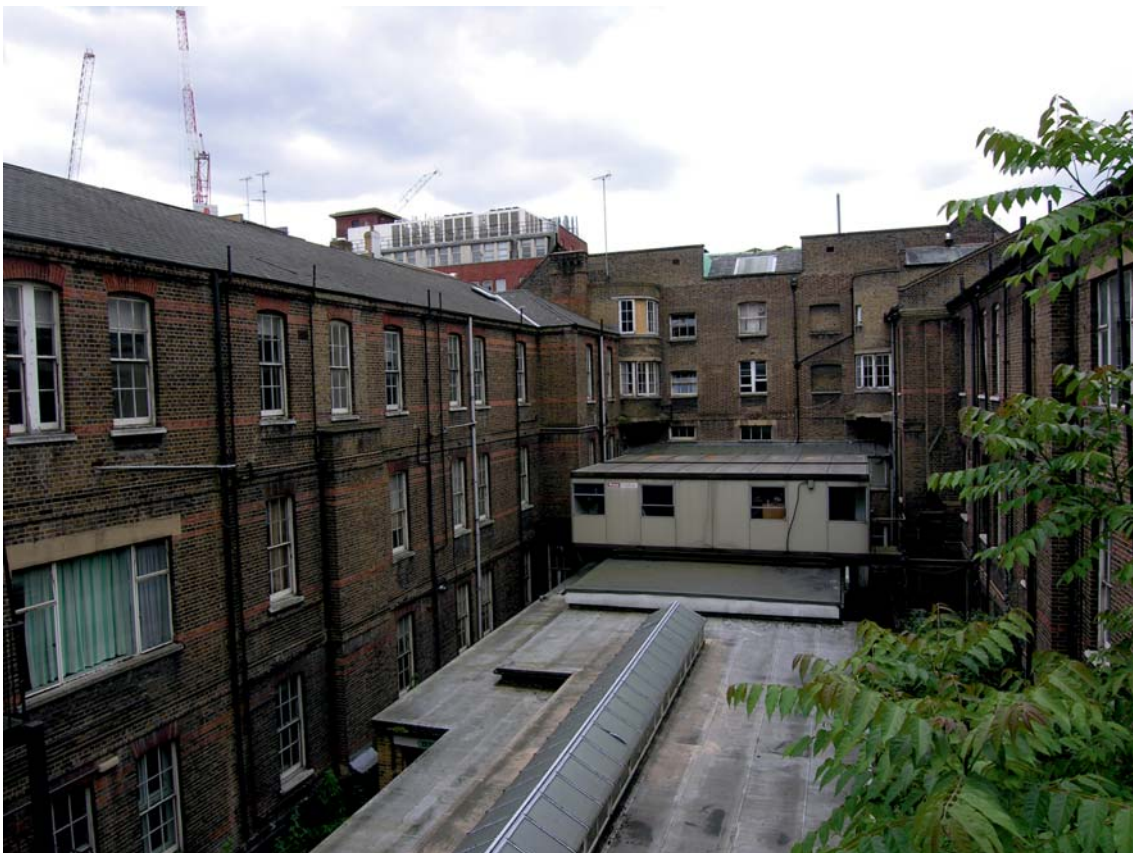
Fig 12 Rear of the late 18th-century building (centre), with two late 19th-century wings extending from its south and north ends, looking south-west (MoLAS 2008)
