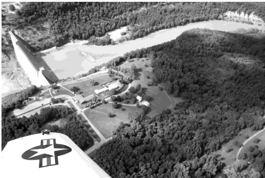
Mt. Morris Dam and FLTC Office
