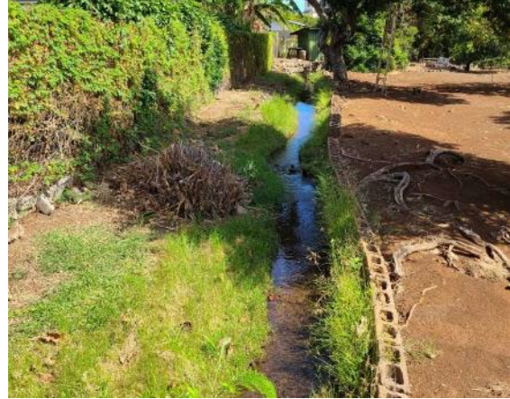
B) Water flows underground from Imua Family Services and drops into an open ditch on the Koeli LLC property.
