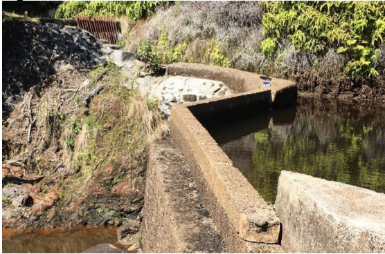
A) Diversion dam at Waiakoali Stream.
