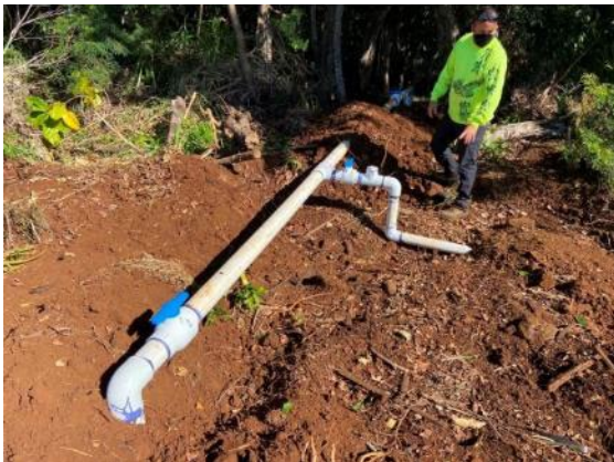
C) Newly installed lateral 4-inch line from Waikapu Properties’ line continues to South Waikapū Kuleana ‘Auwai.
