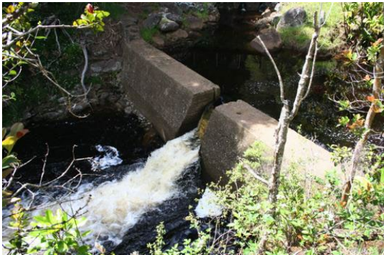
C) Diversion dam at Kauaikinanā Stream.
