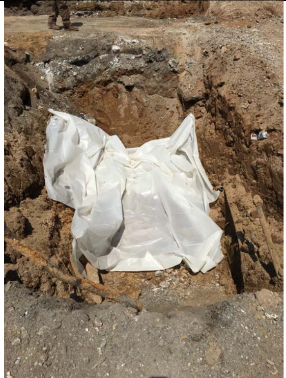
Photo 22: Demarcation layer (i.e. polyethylene sheeting) placed on top of the UST. Photo taken June 22, 2017.
