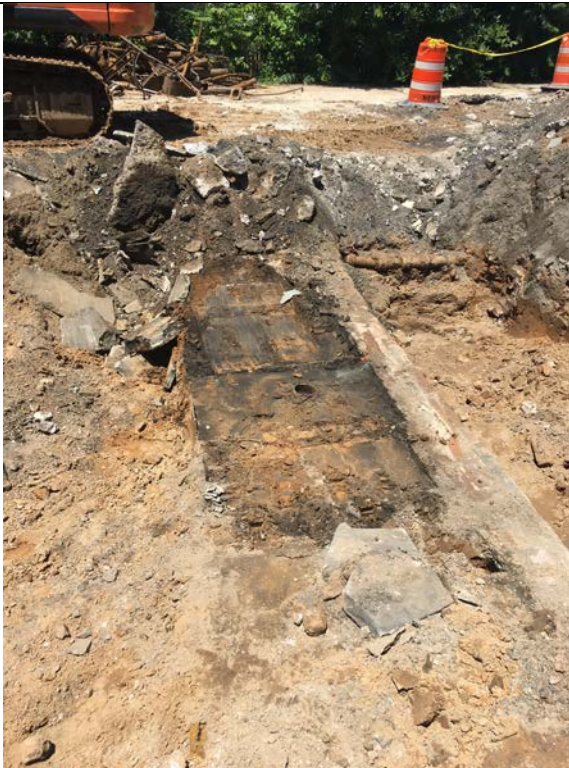
Photo 11: Brown organic soil identified beneath bluestone. Drain noted in center of feature. Photo taken June 20, 2017.
