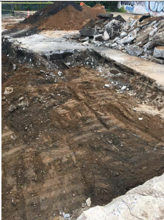
Photo 5: Backfilled portion of Trench 4, taken facing northeast. Photo taken June 16, 2017.
