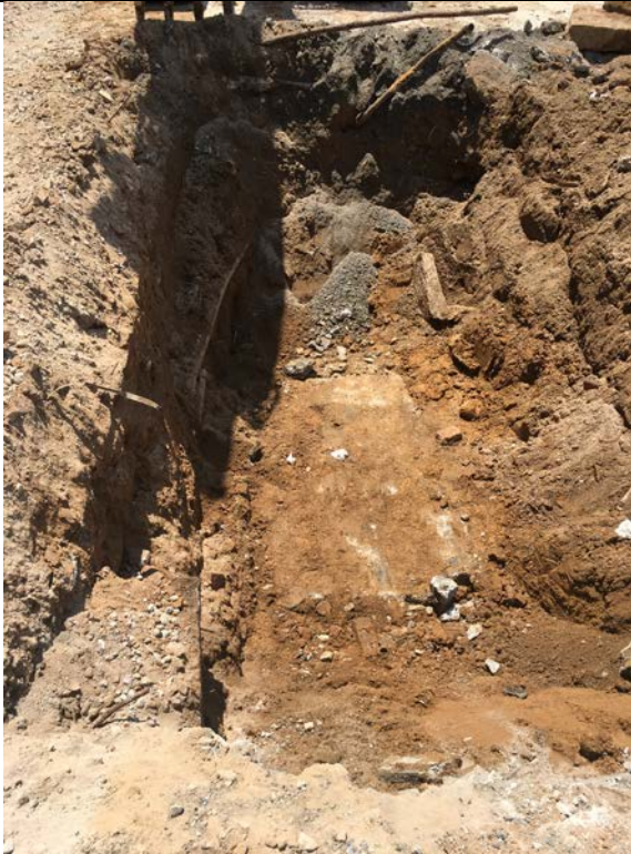
Photo 21: UST identified in Trench 6. Photo taken June 22, 2017.
