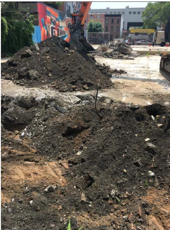
Photo 2: View of soil in Trench 1 taken facing south. Photo taken June 14, 2017.
