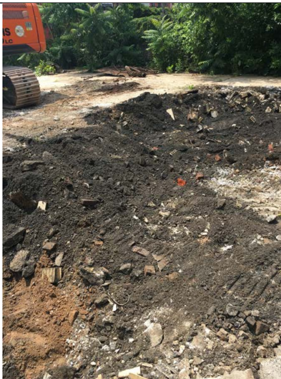
Photo 1: View of soil in Trench 1 taken facing west-southwest. Photo taken June 14, 2017.
