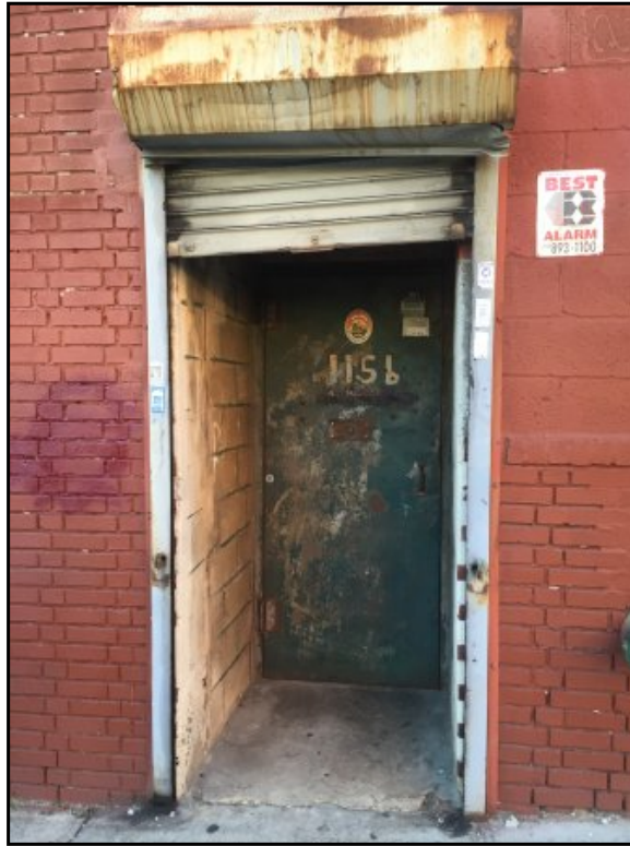
Access to plastic manufacturing facility along 165th Street.
