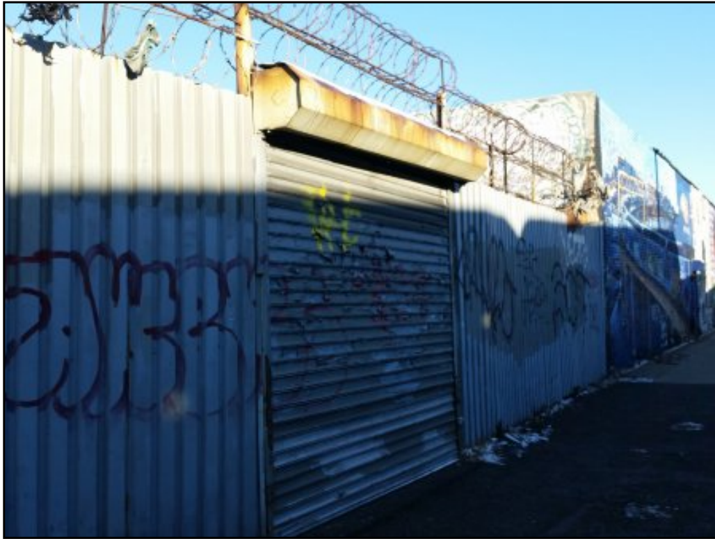
The middle entrance to the storage facility, from Whitlock Avenue.
