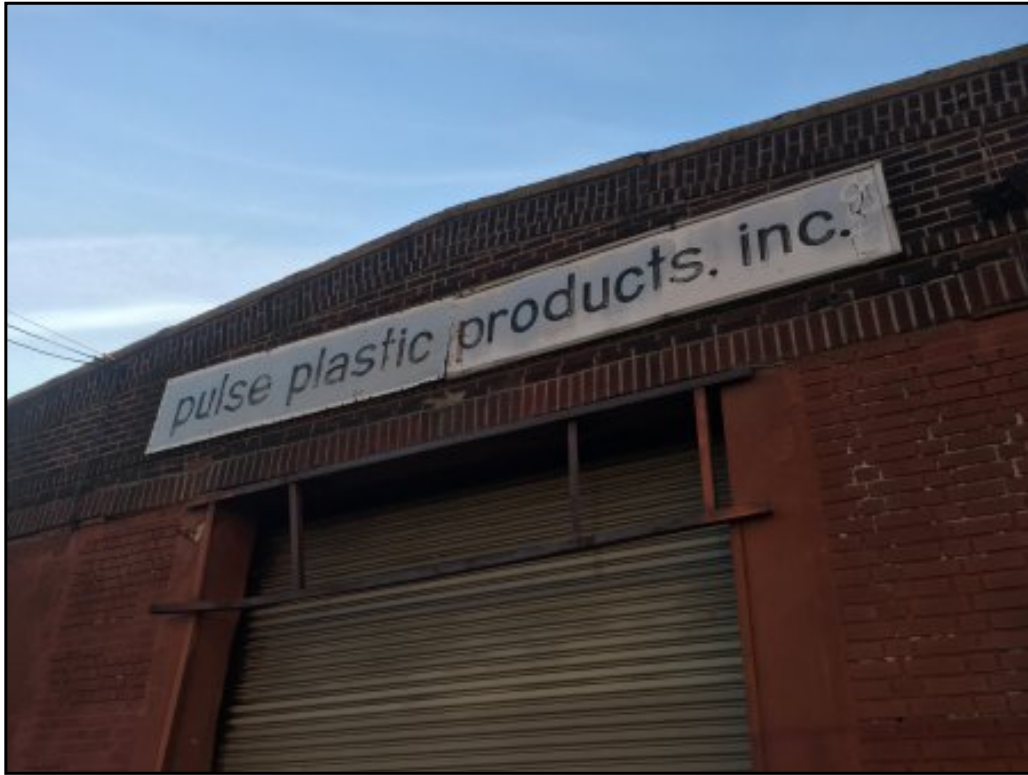
Subject property along 165th Street signage.
