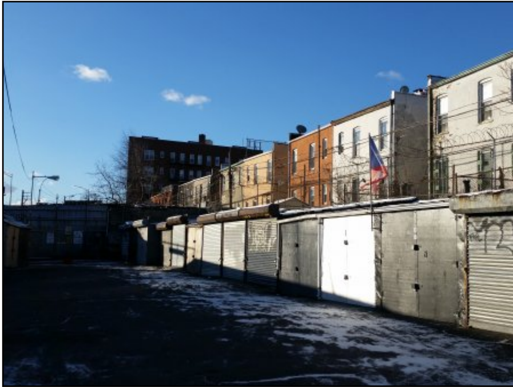
In the central area of the storage facility facing south.
