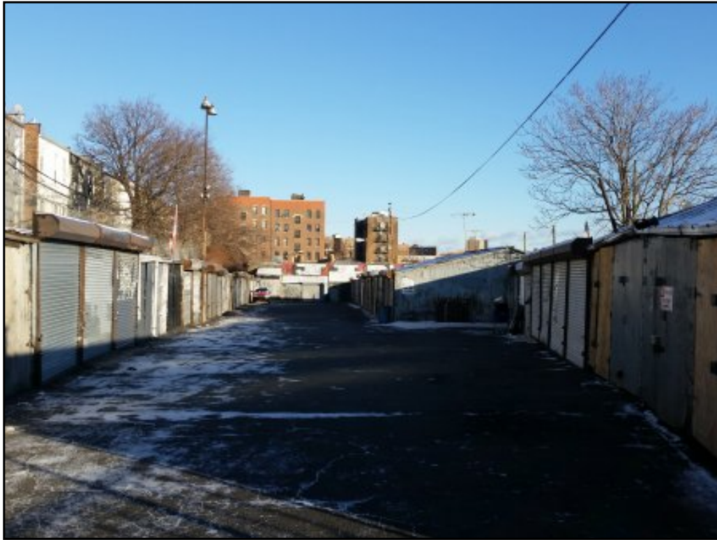
Facing north, inside the storage facility.
