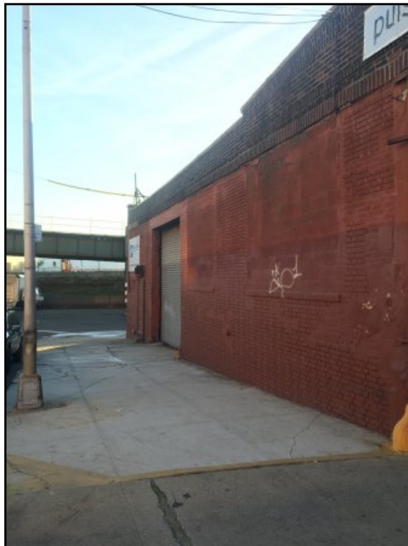
Subject property along 165th Street (facing SE).
