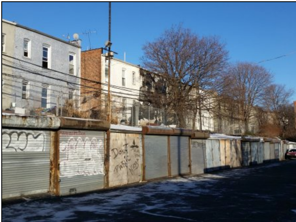
The western section inside the storage facility.
