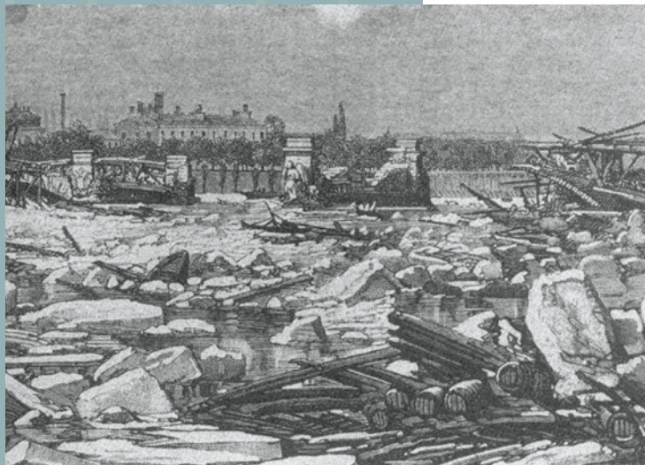
Paris, The Break-up of the Ice on the Seine , January 3, 1880, wood engraving, 1880. The month-long cold spell finally broke on January 3, 1880. As the thaw began and floodwaters rose, large ice floes developed, and piled up against any obstacle in their path. The accumulated ice and debris crashed into bridges with thunderous blows and caused extensive damage. Crowds gathered on the banks and bridges of the Seine to watch as boats, damaged washing establishments, and other flotsam surged downstream towards Vétheuil.
