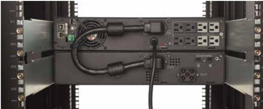
**A UPS paired with an extended battery module helps extend runtime to meet service level agreements.**
