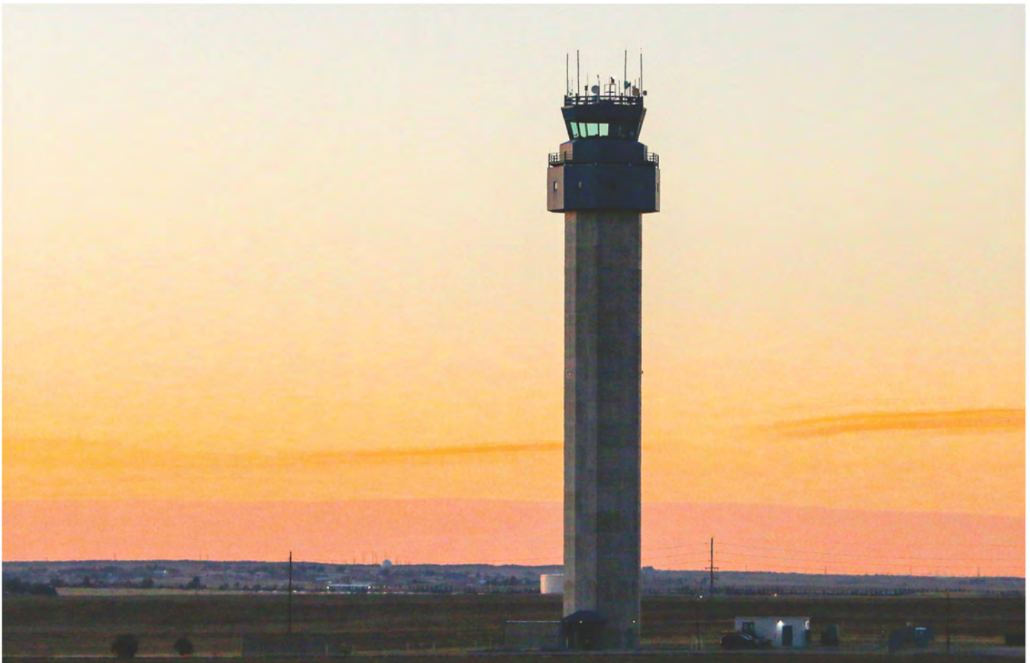
Figure 4-8. CASP Air Traffic Control Tower
