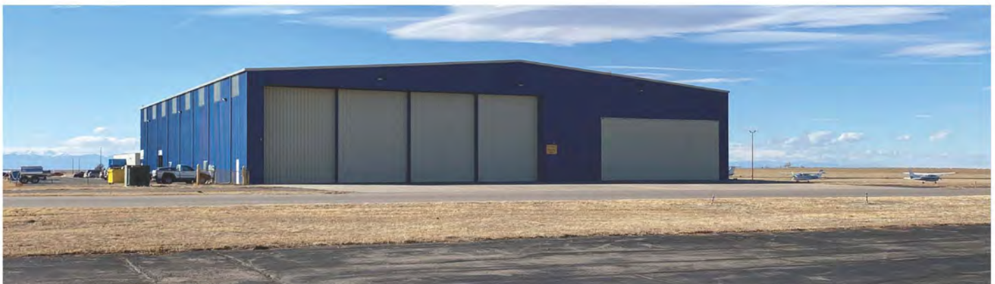
Figure 5-8. Existing Hangers at CASP
