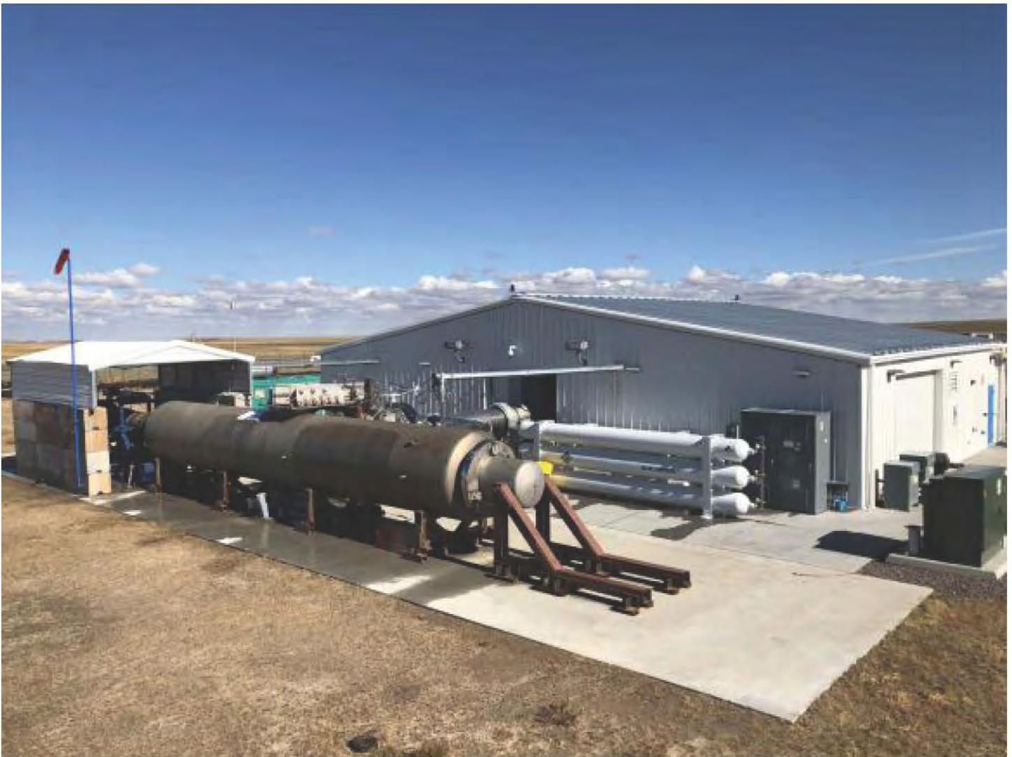
Figure 2-5. Reaction Engines Test Facility 2
