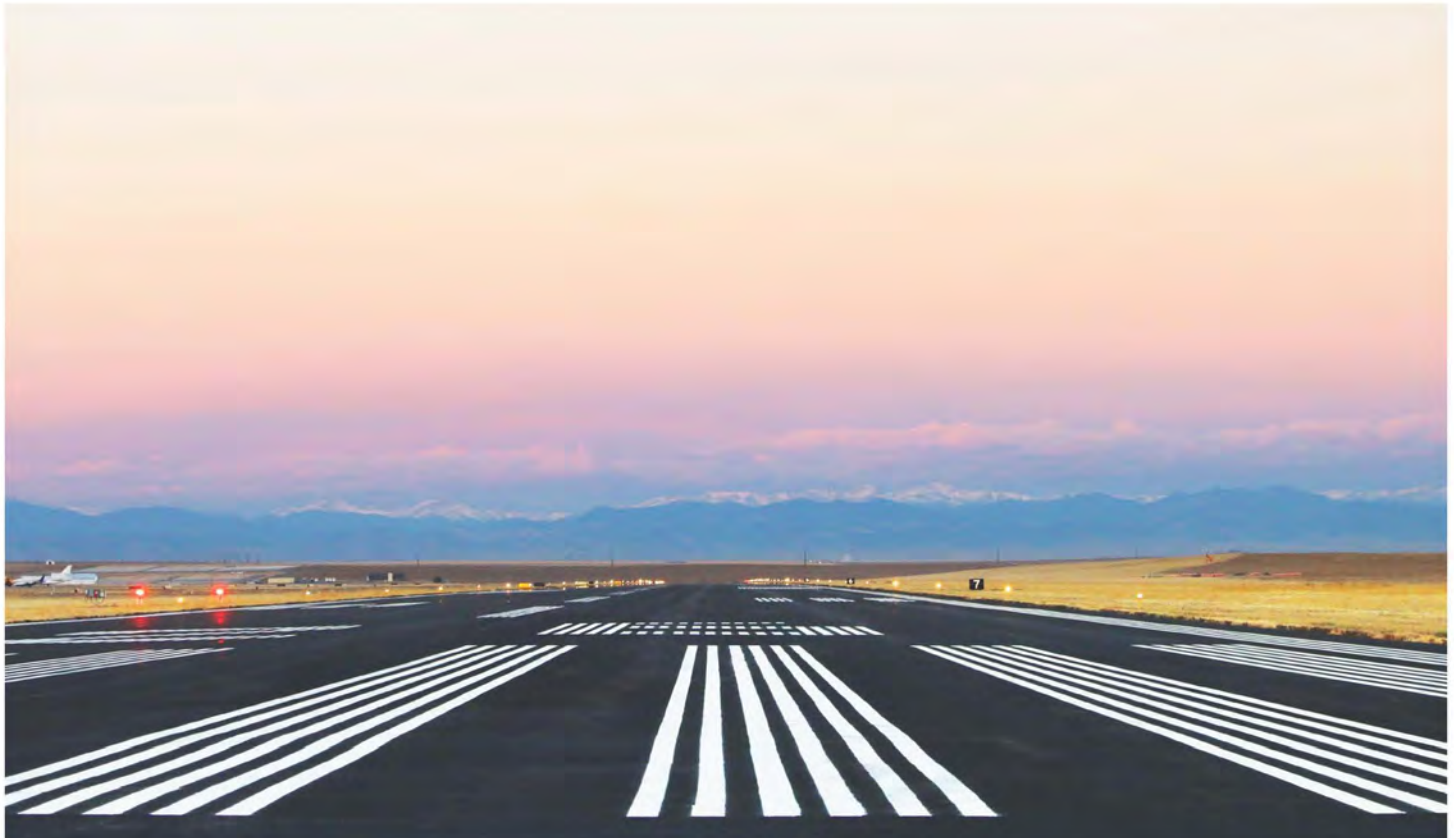
Figure 4-2. Runway 26 Looking West at Dawn
