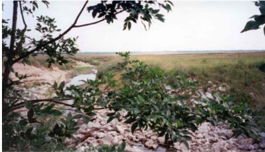
Looking north at Bonnie Creek, riprap and other bank stabilization efforts are visible.
