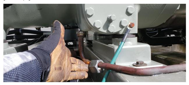
Figure 18. Fitting installation for suction transducer in the suction line
