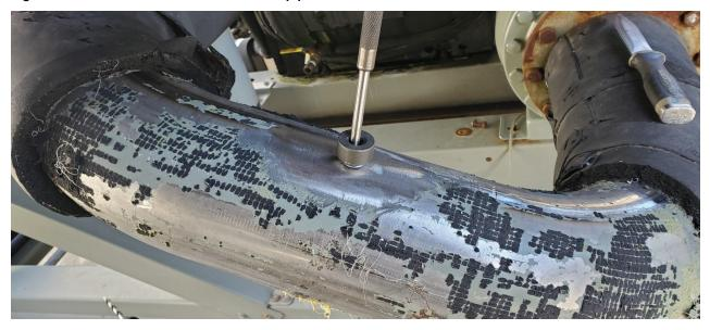
Figure 20. Follow standard welding procedures when welding 1/4 inch pipe thread threadelet in place
