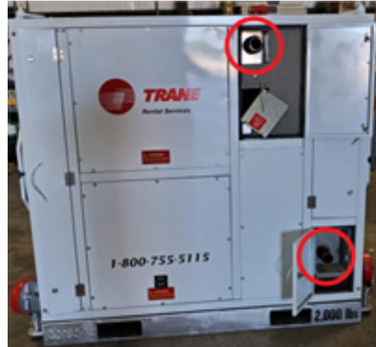
Figure 38. RSAU0010F0 - Victaulic water lines
