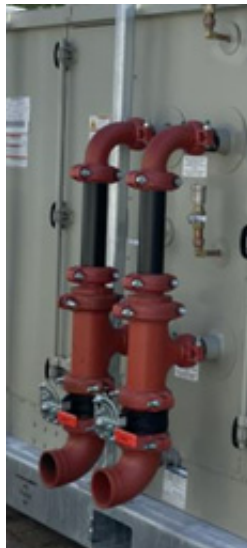
Figure 42. RSCC0030F0 - Manifold coil connections
