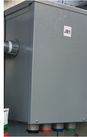
Figure 33. Series 16 cam type electrical connections
