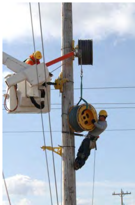
Idaho Power linemen install upgrades.
