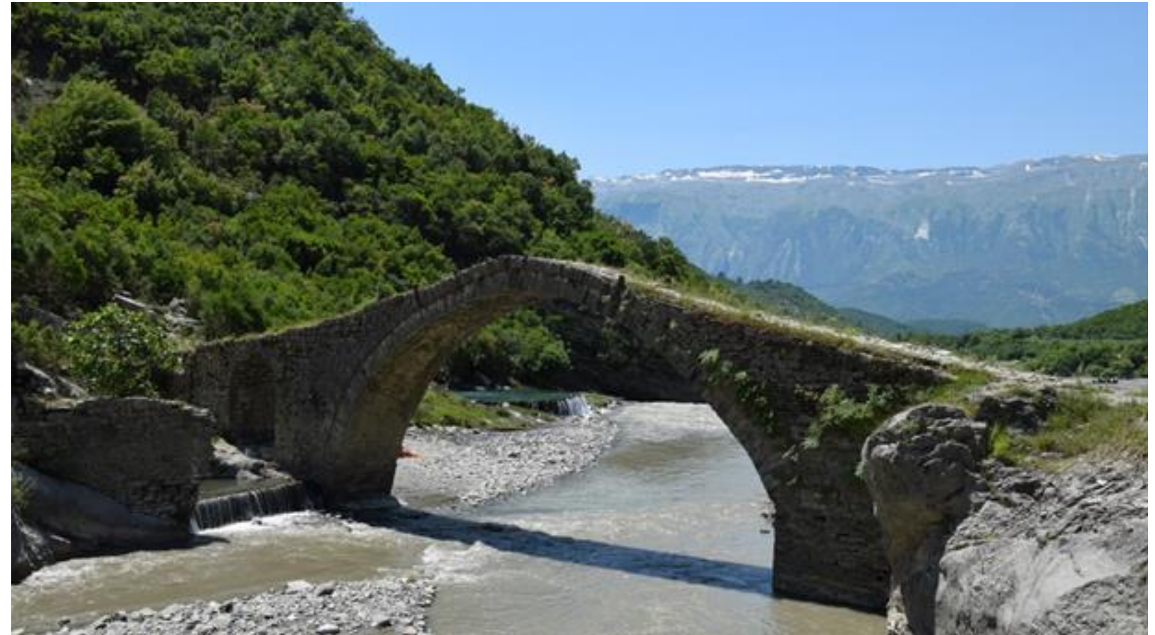
Katiu bridge in Bënja: Historical monument of ottoman period
