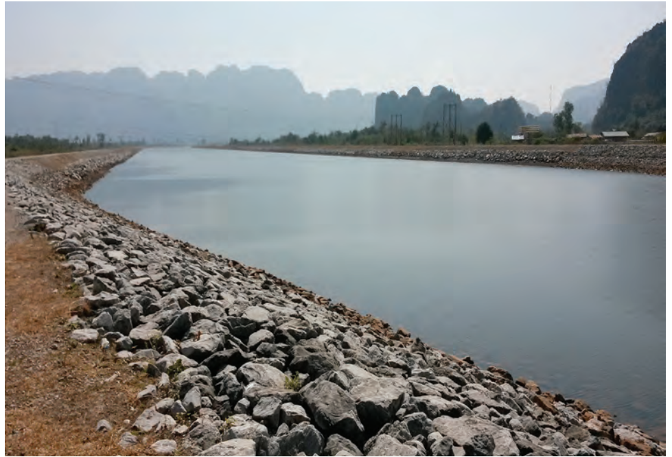
NTPC discharge channel downstream
