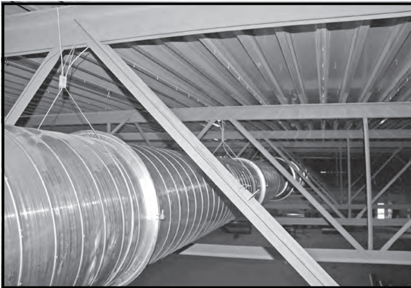
Installed CL23-WC6 Cable Locks
