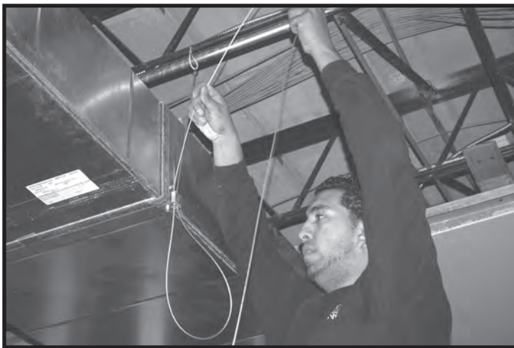
Installation of the KV Bracket at the Elmont Library in Nassau County, NY
