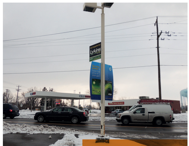
Figure 34: Permanent light pole with temporary sign components.
