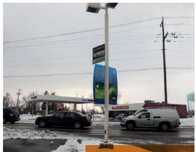
Figure 34: Permanent light pole with temporary sign components.
