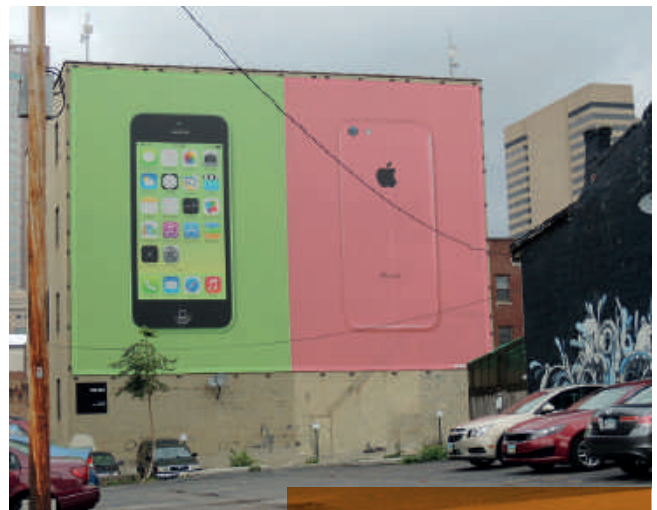
Figure 21: Example of a temporary advertising mural attached to a blank building façade.
