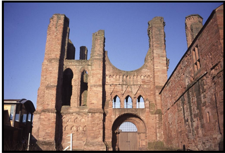
Figure 7: west front of the abbey, showing the remains of the two western towers. That on the north (left) was apparently heightened following damage in the late thirteenth century (collection of R Oram).
