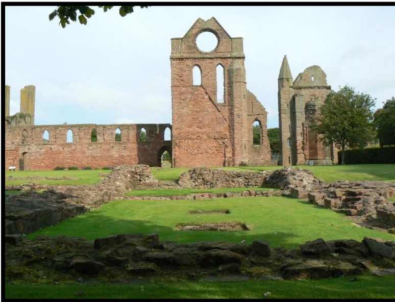
Figure 9: looking N along the site of the east range of the cloister towards the south gable of the south transept. The dormitory occupied the upper floor of this range and the high pitch of its roof can be seen fossilised in the lower half of the gable. A door at this level entered the night stair down which the monks processed to their choir for the night offices (collection of R Oram).
