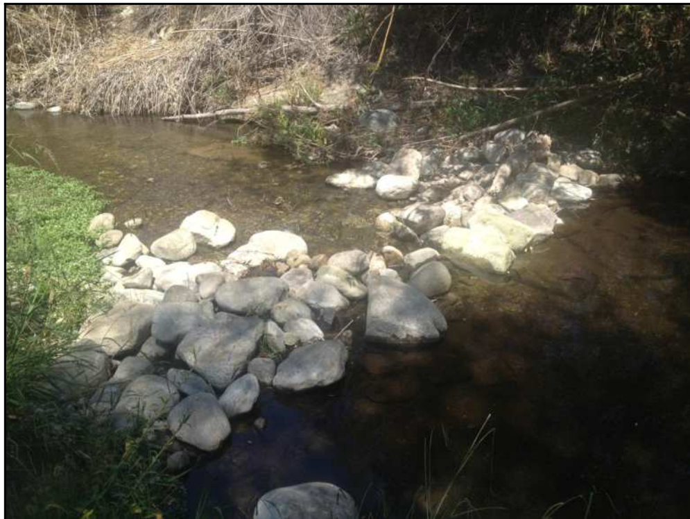
Figure 2. Rock dam blocking the natural flow of Haines Canyon Creek on August 25, 2013.
