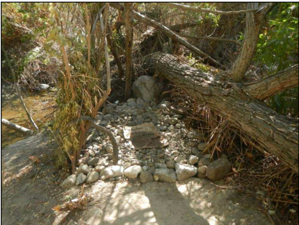
Figure 6. Inside the shade structure near second picnic area.
