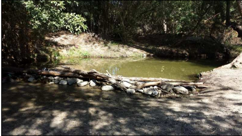
Figure 3. Large Rock Dam present at the popular swimming area near the South Wheatland entrance on September 1, 2013 (Labor Day Weekend).
