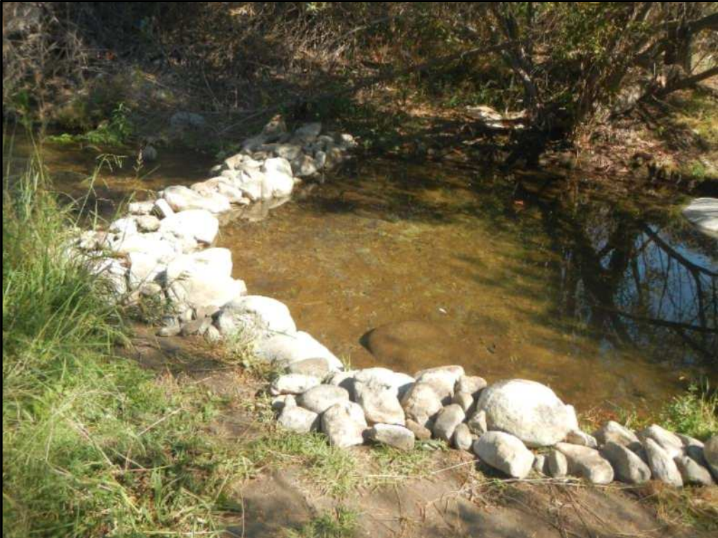
Figure 4. Rock dam within Haines Canyon Creek at the second picnic area.
