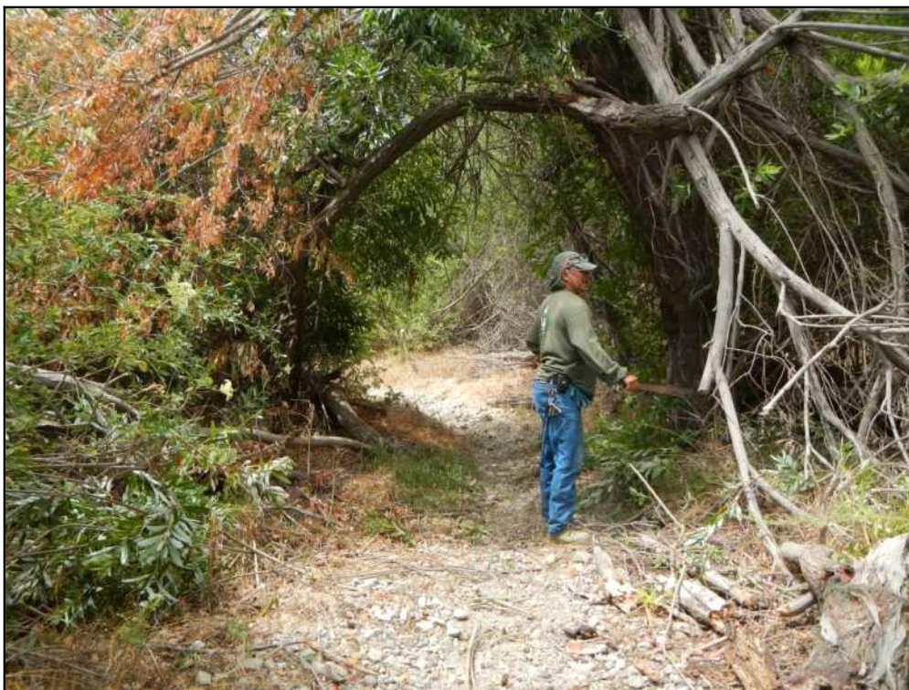
Figure 2. Crew clearing vegetation along trail.
