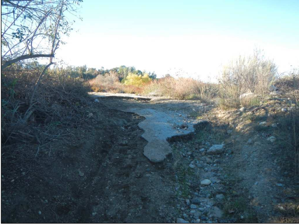
Figure 5. Eroded trail between Cottonwood upland area and Haines Canyon Creek.
