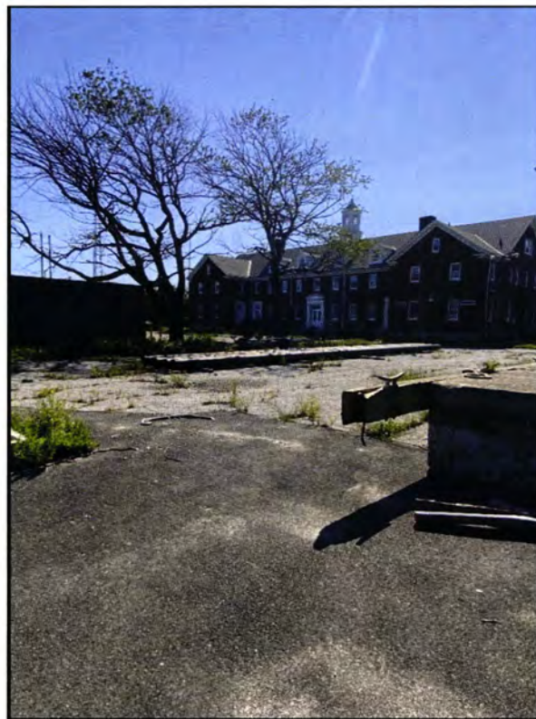
Photo 6 - View of upland area behind bulkhead.
