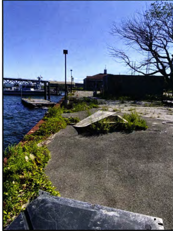
Photo 5 - View of project site, dock and bulkhead, looking east from bulkhead Sta. 2+10.
