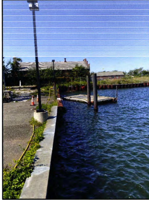
Photo 3 - View of project work zone, looking west from bulkhead Sta 3+70
