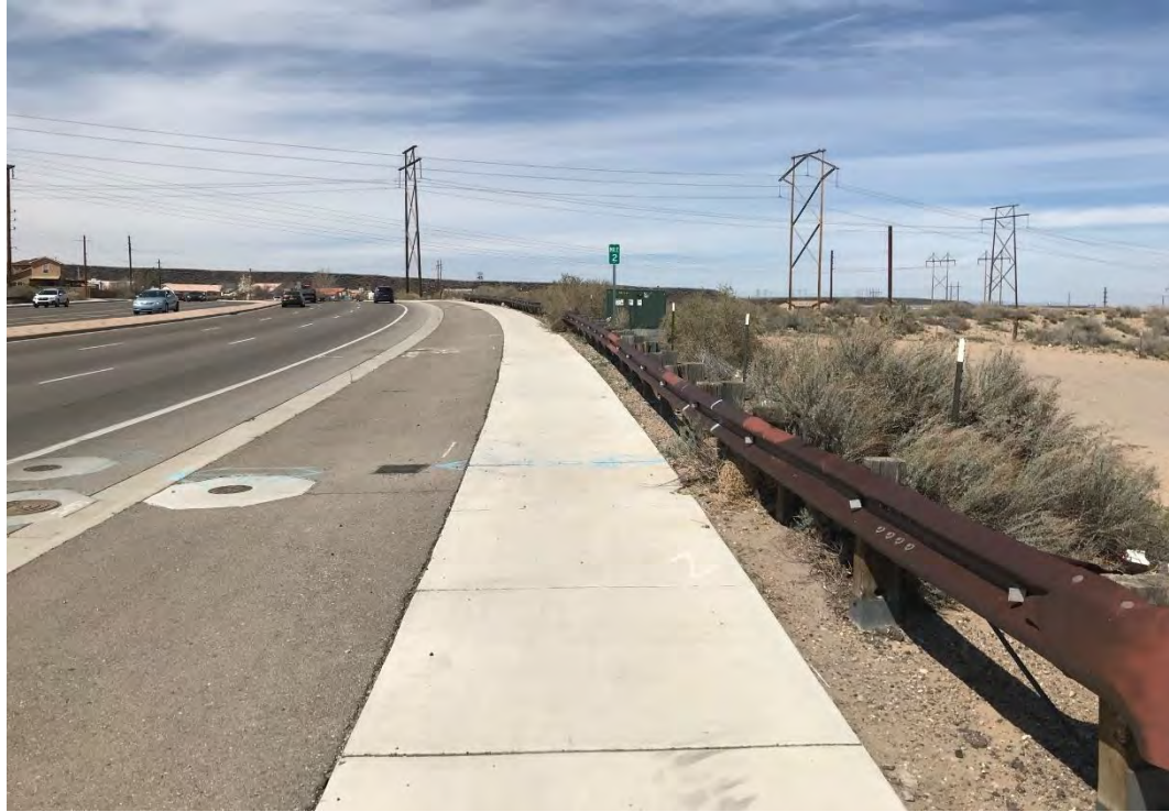
Figure 7: Looking north along west edge of site (Unser on left) showing existing sidewalk and guardrail that will remain.
