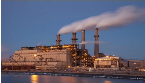
San Juan Generating Station Farmington New Mexico
