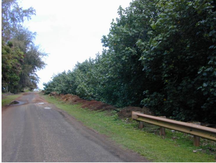
Photo looking makai along Hilton Lane. The drainage ditch is to the right of the road. Earth and debris from recent ditch cleaning can be seen along the ditch. The proposed culvert path crossing is located approximately 25 feet past the end of the guardrail.
