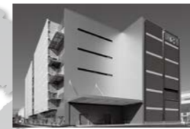
Industrial Mechatronics Systems Works/ Nagoya Works
