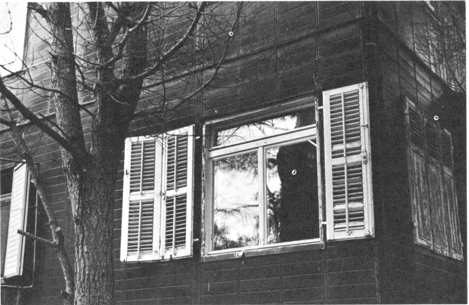
4.6 Hirsch Kupfer-und Messingwerke, window detail, copper houses (Grundman House, Haifa, 1933–34, by Deutsche Kupferhaus Gesellschaft).
