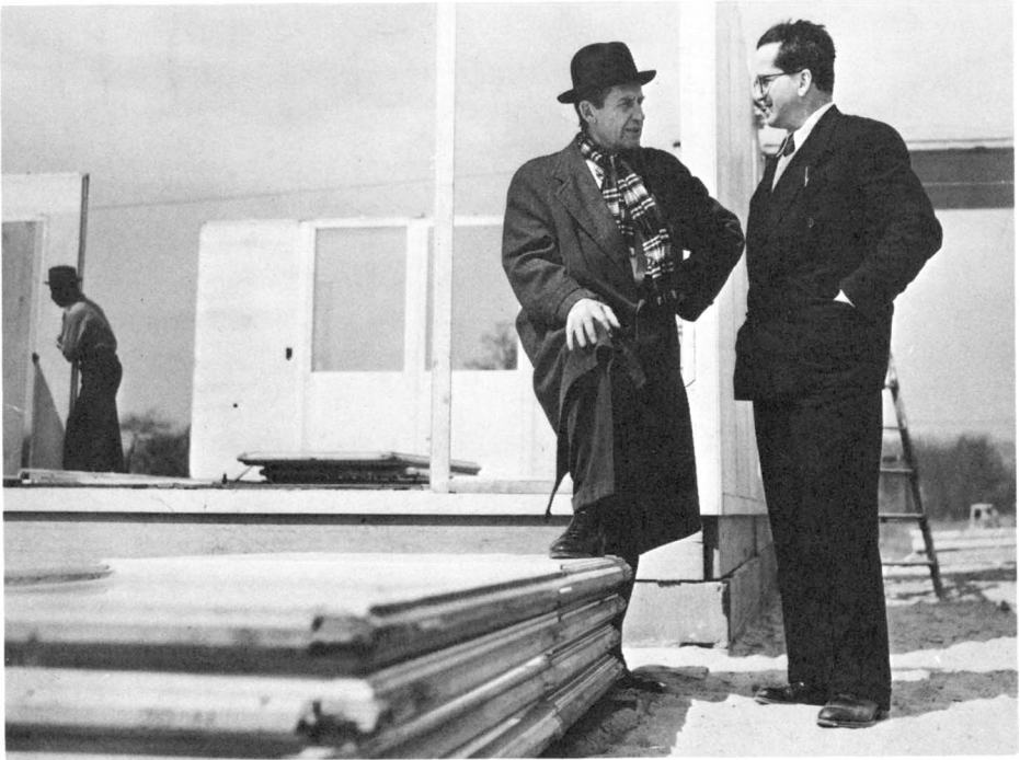
9.9 Walter Gropius and Konrad Wachsmann, inspecting test house, General Panel, Queens, N.Y., 1946
