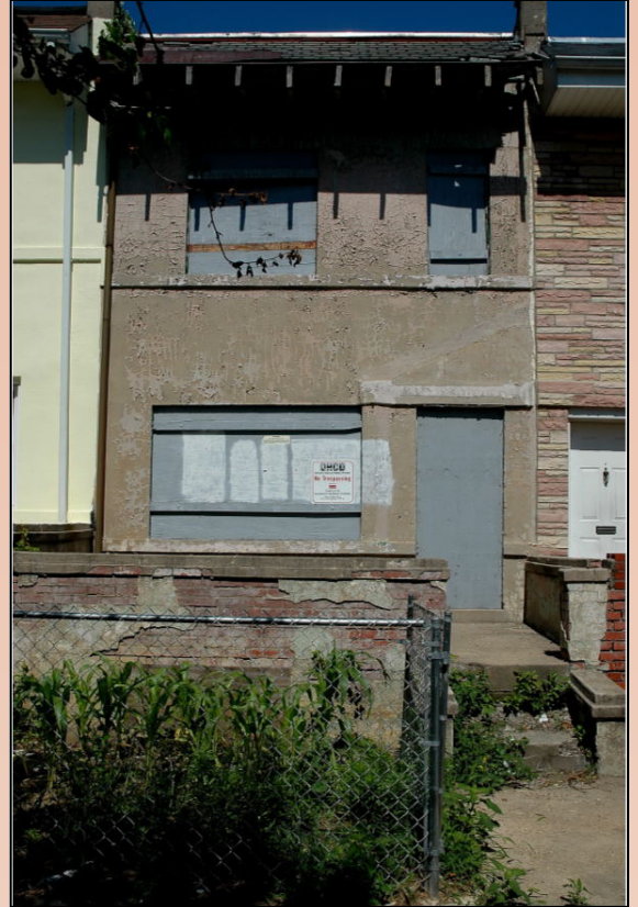
Auctioned Property: 3620 Rock Creek Church Rd., NW
