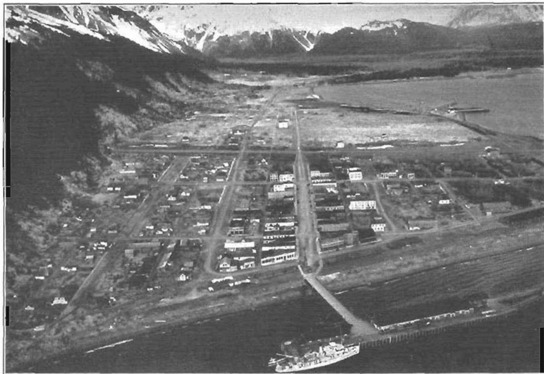
AIR VIEW OF SEWARD, THE COASTAL TERMINUS OF THE ALASKA RAILROAD.
