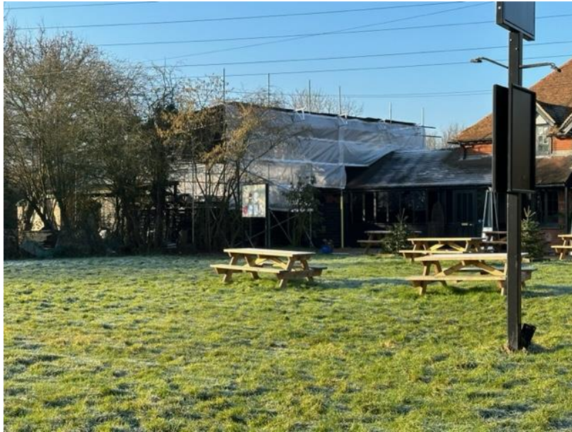
Figure 1: Photograph of unauthorised structure within outdoor seat area of Tranquil Turtle.
