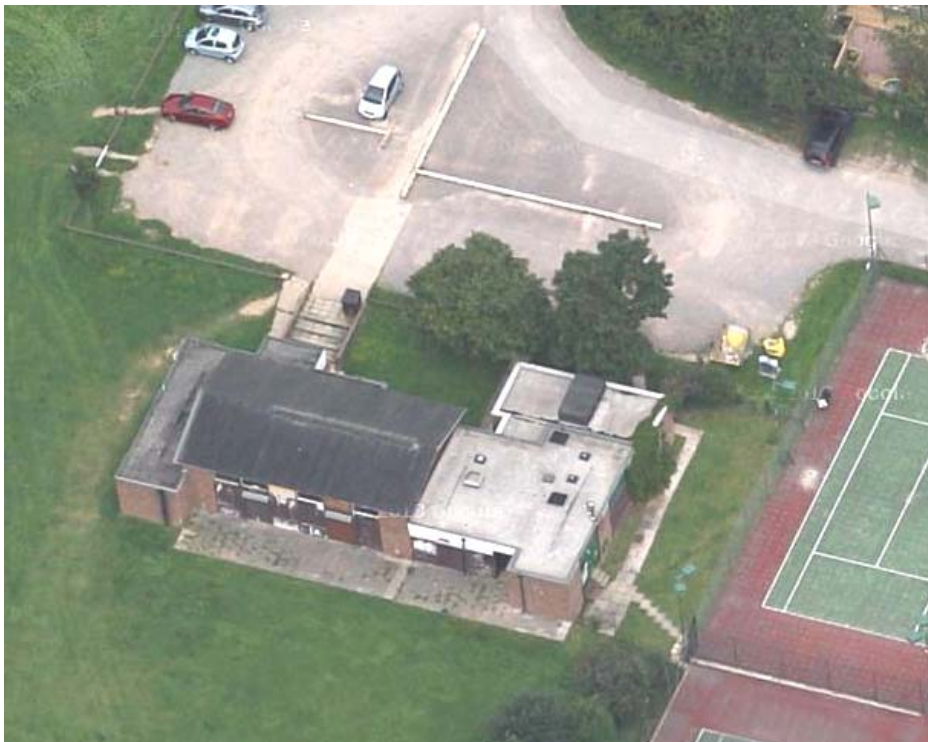
Figure 1.2 Existing building viewed from the south
