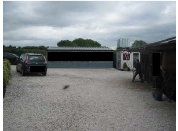
(The replacement kennel building pre erection of the acoustic fence)
