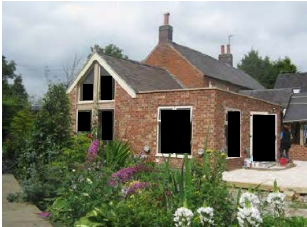
(The Existing Dwelling at Four Lane Ends Farm)
