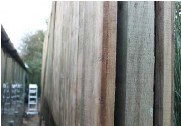
(Fence construction - close boarded with a mineral wool insulation core)
