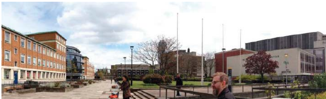
Image 3: site prior to partial demolition and hoarding
