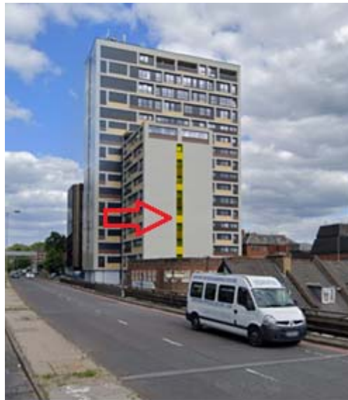
Fig 17 – Location of major VSC ratio failures on Impact House
