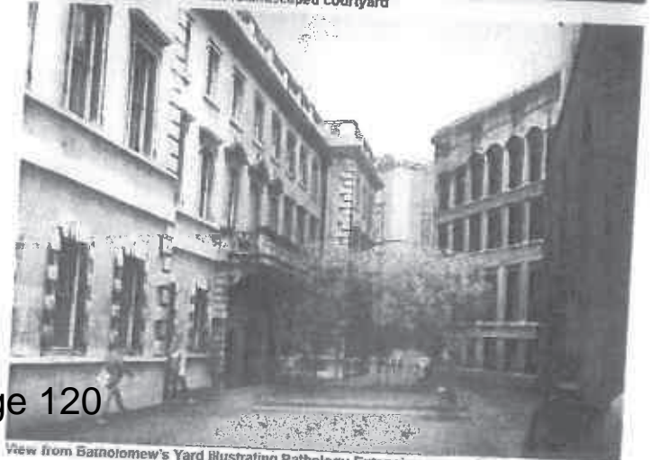
View from Bartholomew's Yard illustrating Pathology Extension removal
