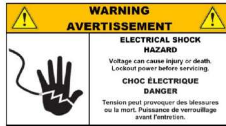
LOCATED ON: DRYER CONTROL CENTER
