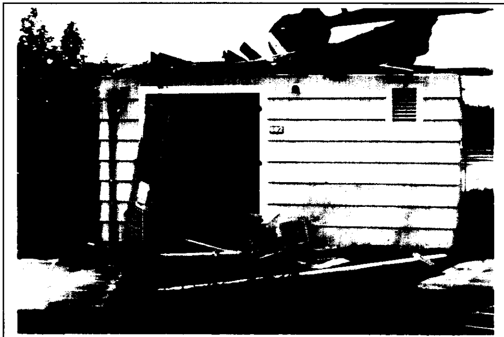
Photograph 9-6. Building 602 demolition, facing south.
