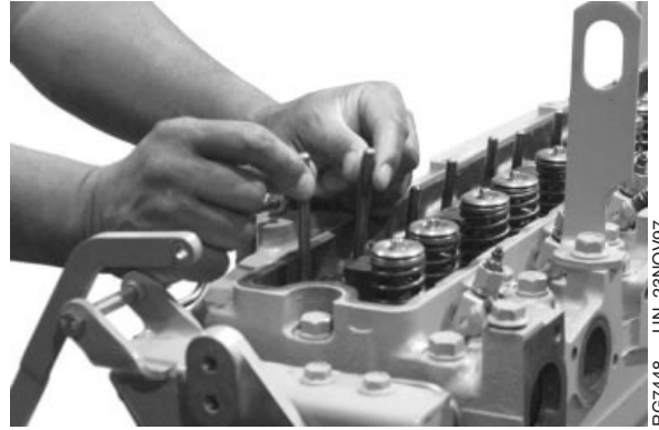
Rocker Arm Assembly Installation
