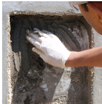
Moist cure and protect from elements immediately after finishing.
