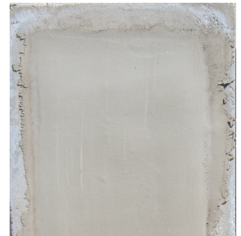
Finish with trowel, float, or sponge, depending on desired surface texture.
