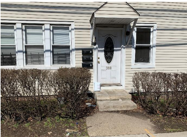
Front of building.
