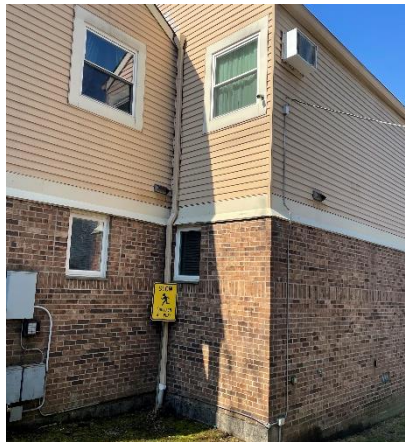
Side of condominium building.
