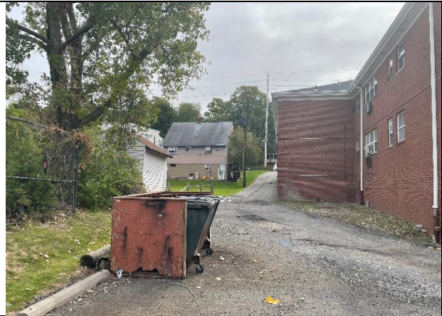
View from the rear of the site looking towards Grand Avenue and the driveway. There is a substantial drop in the westerly direction.
