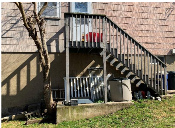
Side of building.
