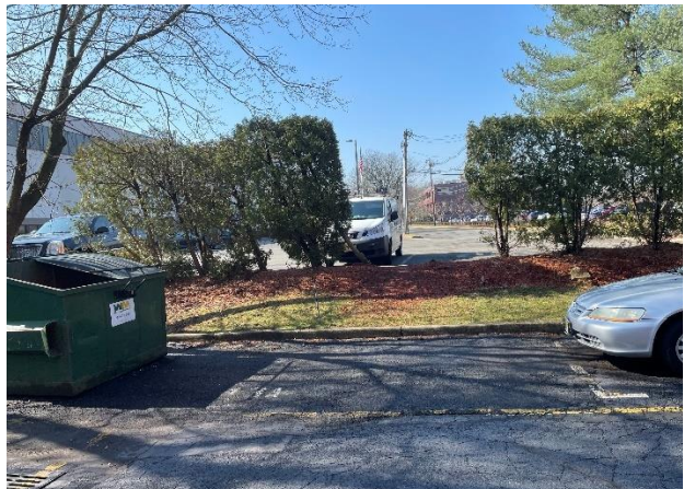
Inadequate parking space layout. Unscreened waste container.
