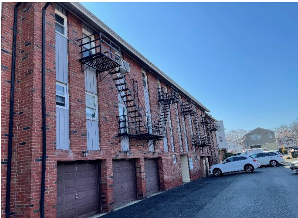
Rear of building with exposed fire escape and cars parked in the driveway leading to the garage.
