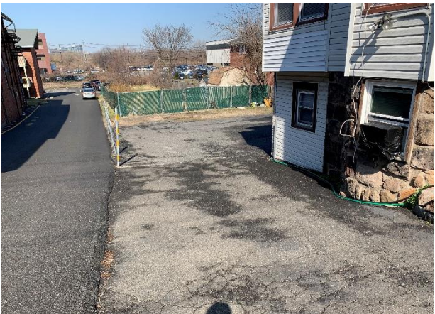
Access to rear parking area showing the narrowing of the driveway. Exposed window A/C unit.
