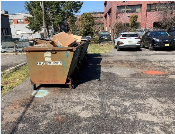
Exposed trash container with lack of screening. View looking towards the westerly property line
