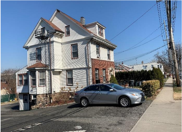
Triplex fronting Grand Avenue. Exposed fire escape.
