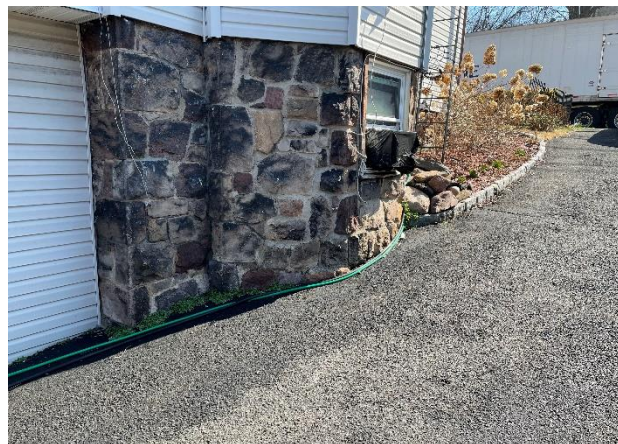
View from the rear looking towards Grand Avenue showing the drop in topography and the trailer standing to make a turn on to Fort Lee Road.
