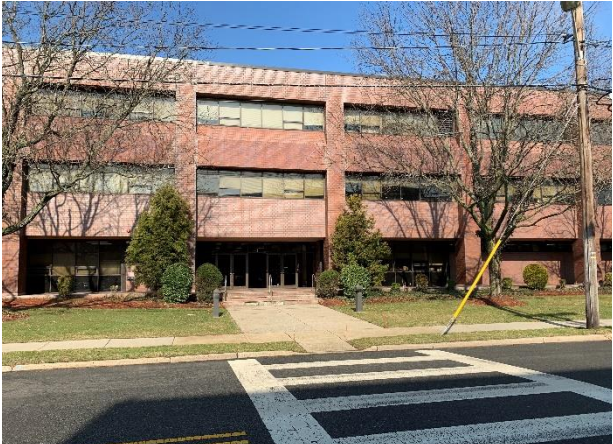
Side of building.
