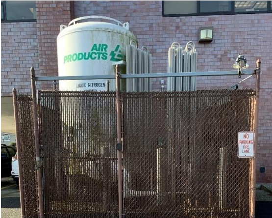
Enclosed liquid nitrogen container.
