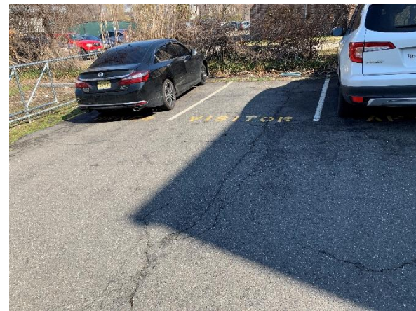
Rear parking area with striped parking spaces.
