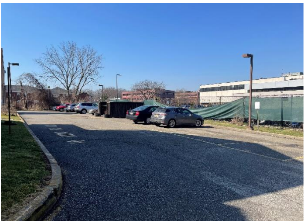
Rear parking lot.
