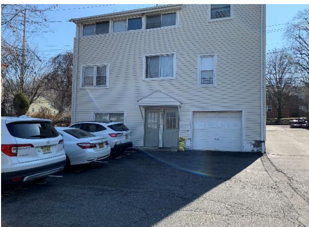
Rear of structure. Parking area and parking access.
