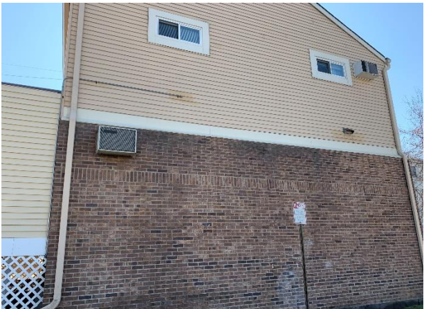
Rear of the condominium building with exposed A/C units.
