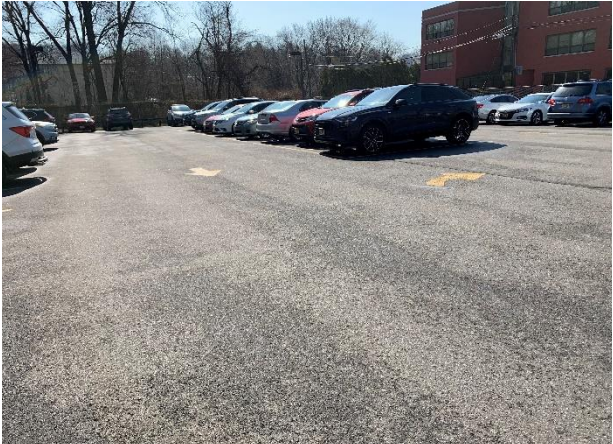
Existing parking lot.
