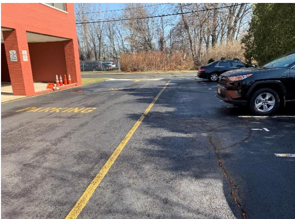
Egress from parking lot onto Schor Avenue.
