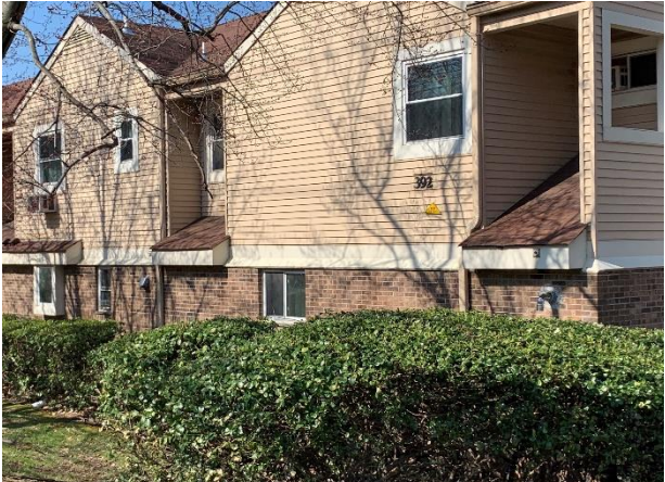
Dwelling fronting on Grand Ave. Window A/C units for each condominium.
