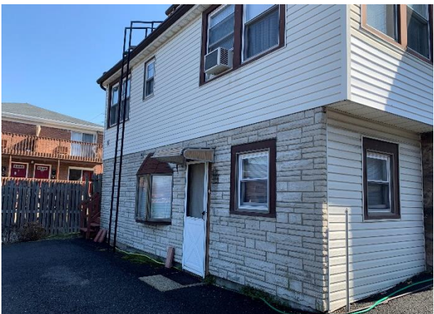
Rear of structure. Walkout basement and window A/C units. Parking area flush with the rear façade of the building.
