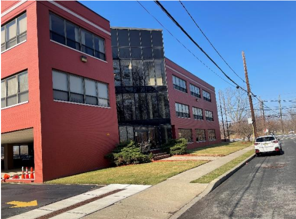
Front of office building fronting on Schor Avenue.
