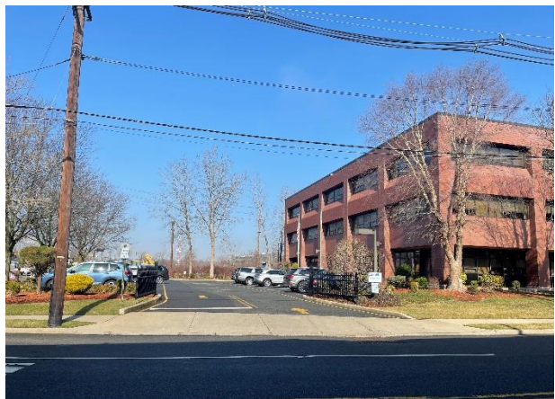
Front parking lot.
