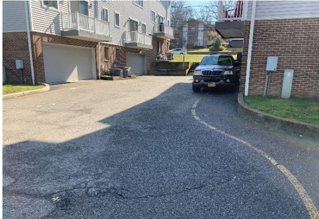
View from the entrance driveway looking towards Grand Avenue
