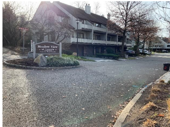
Townhome development on Station Parkway
