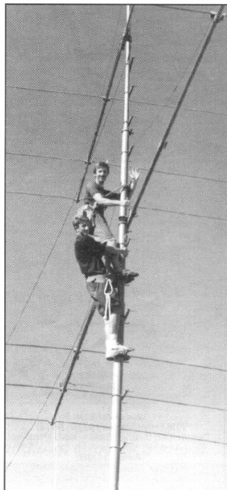
Wes, SP4EEZ (SP4Z), up the tower with his brother placing the homebrew 6-element Yagi on the mast.
