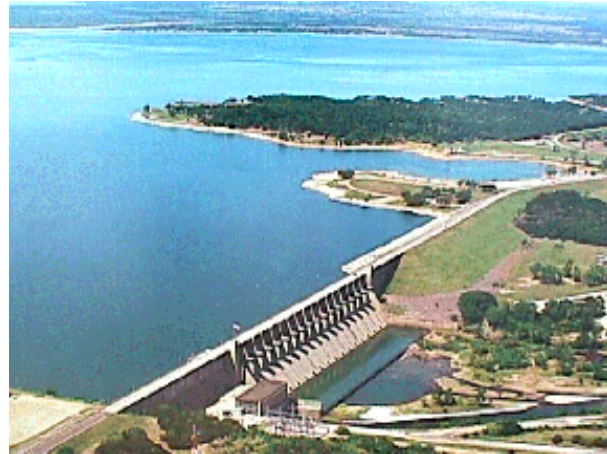
Whitney Lake outlet structure and powerhouse
