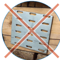
Double stringers, patched boards, or metal repair plates are NOT ALLOWED .
