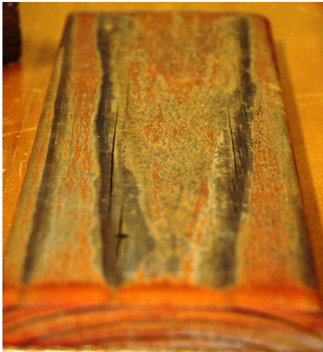
Figure 2.5: Image of a tangentially cut board, containing a film forming finish which was weathered for 1 year.
