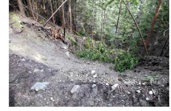
Photo 2. Landslide paths below resource roads
