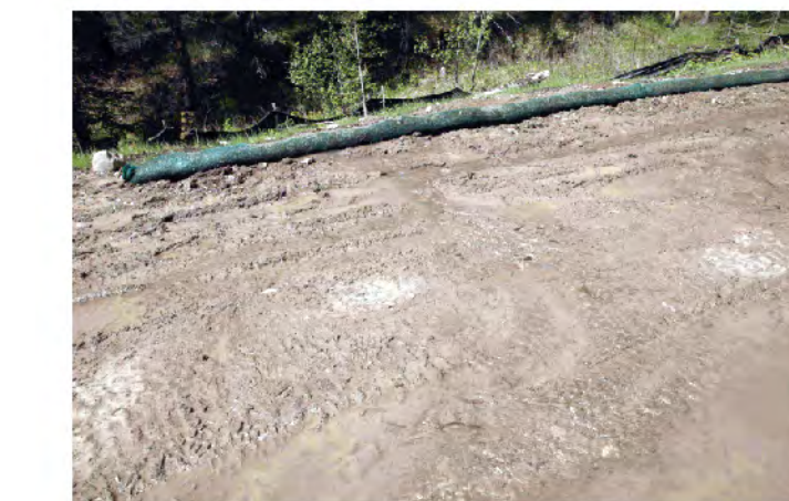
Photo 2. Erosion from road surfaces
