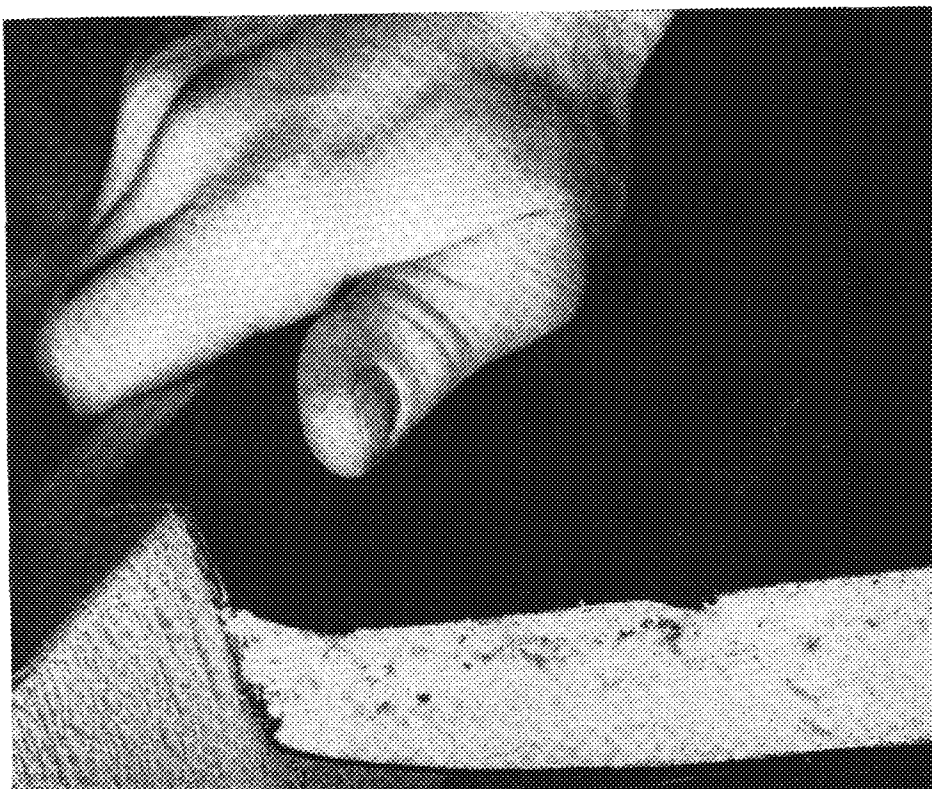
Closeup of ceiling installation
