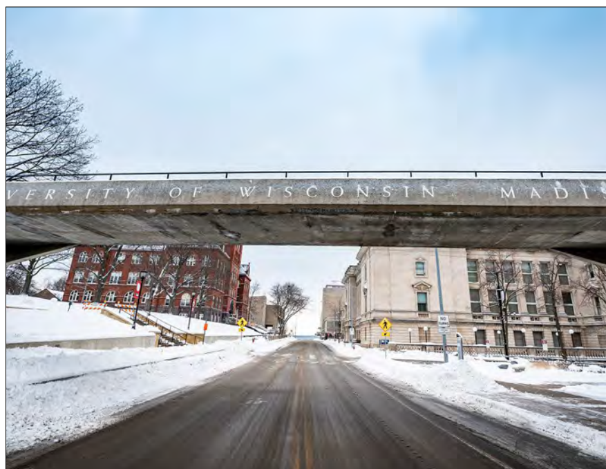
Park Street pedestrian bridge
