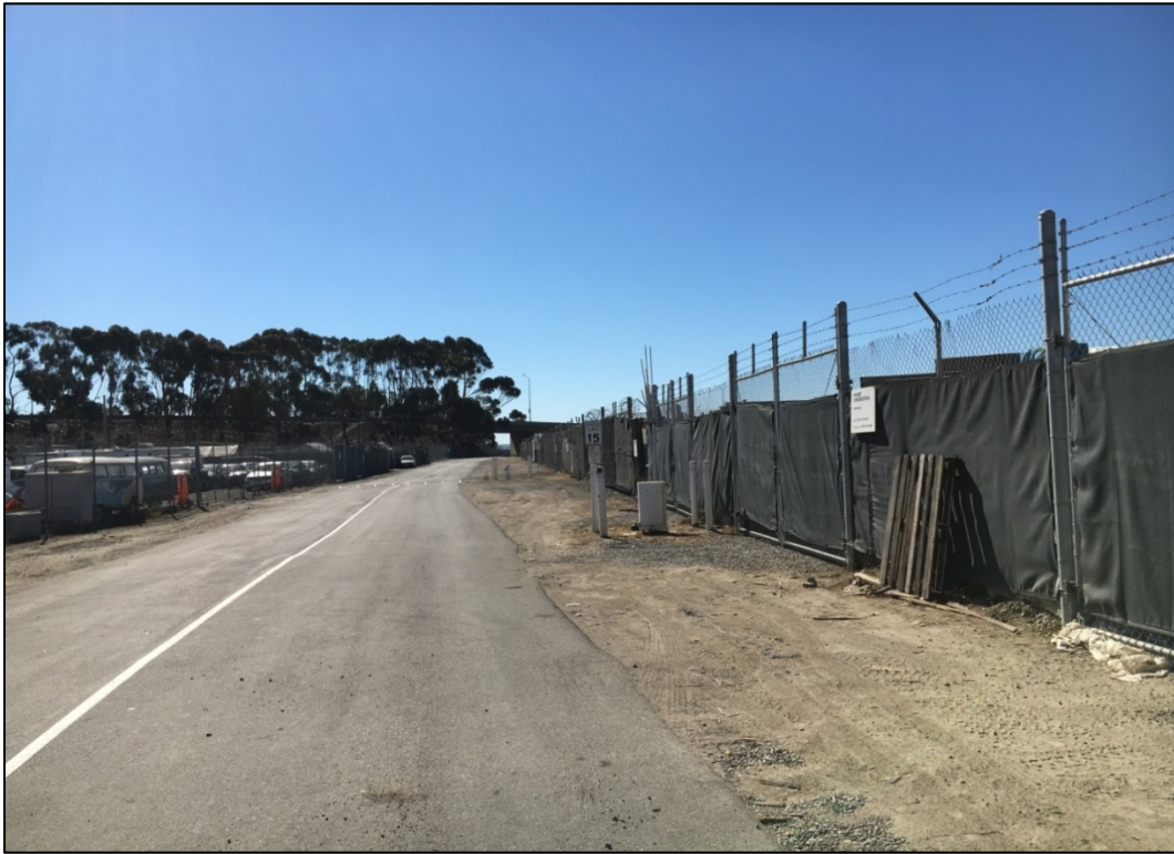
Photograph 1. View of paved and fenced portion of South Site, facing south.
