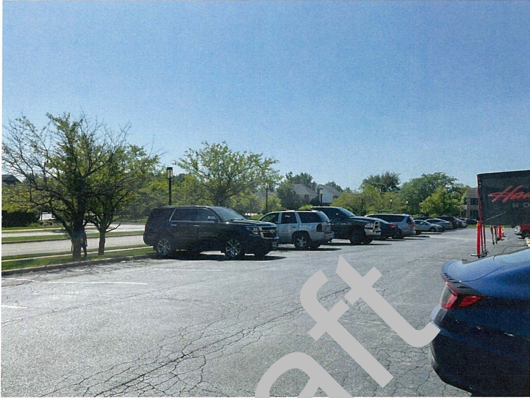
View of parking lot looking south east.
