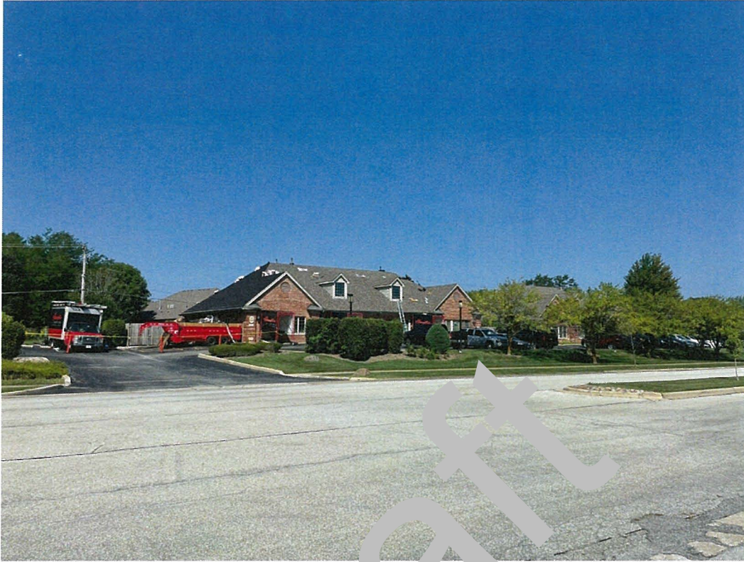
View of ingress/egress site looking northwest.
