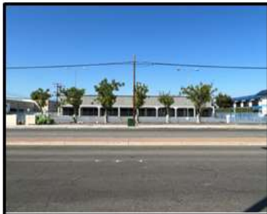
Photo 5: South view of project site looking north from Lincoln Avenue to the project site.
