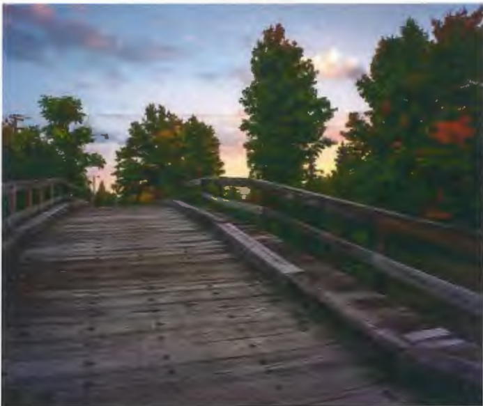
Isbell Street pedestrian bridge
