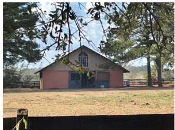
VIEW OF CONCRETE BLOCK HORSE BARN
