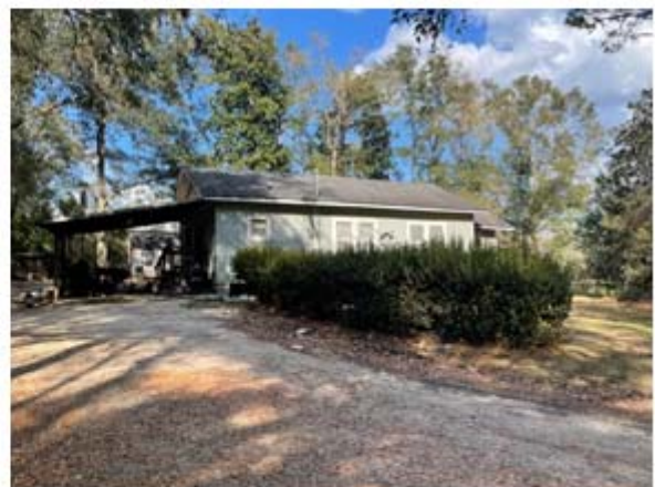
SIDE VIEW OF SF RESIDENCE
