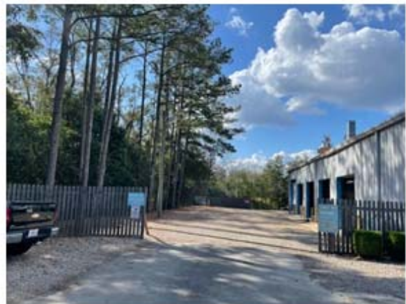
VIEW OF SOUTH PARKING/DRIVE AREA OF SHOP
