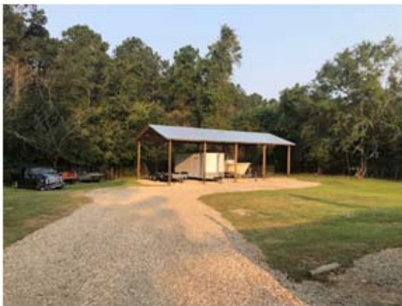
VIEW OF TENANT-OWNED POLE BARN AT BODY SHOP
