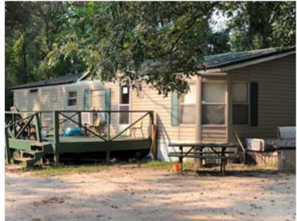
VIEW OF SOUTH MOBILE HOME- HOGAN LANE
