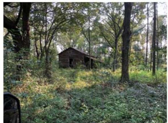
VIEW OF NORTH PORTION OF AG-ZONED LAND (AND DILAPIDATED BARN)
