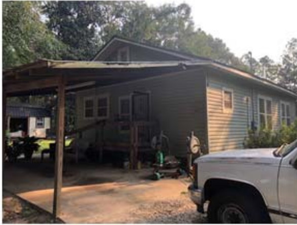
REAR VIEW OF SF RESIDENCE
