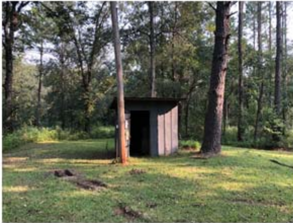
VIEW OF WELL HOUSE
